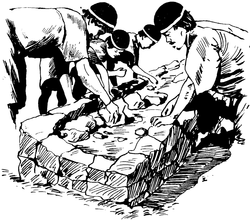
Laying the foundation of a house
